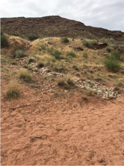
Erosion Structure on BLM Near Mill Creek
