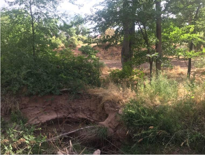
Erosion near Walker Street in Moab
