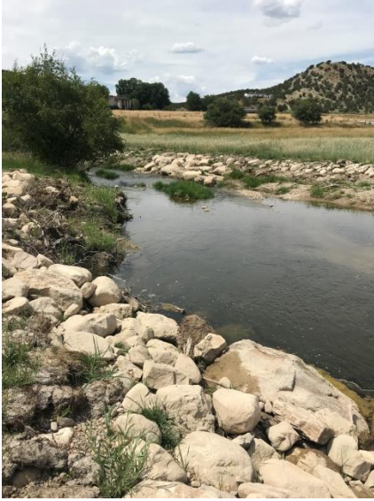
Carter Stream Bank Stabilization Project
