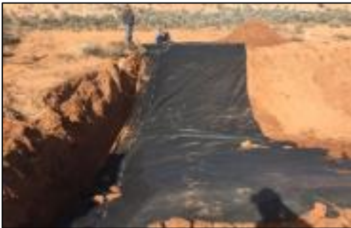
Geo-Fabric was installed (Shown) and covered overlain with riprap.
