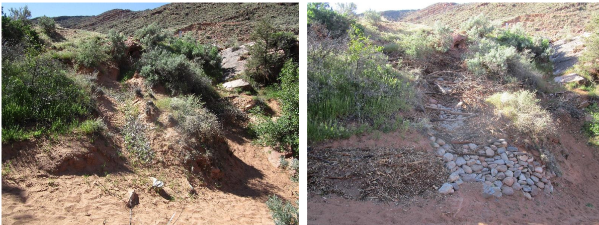
Before/after gully control structure construction
