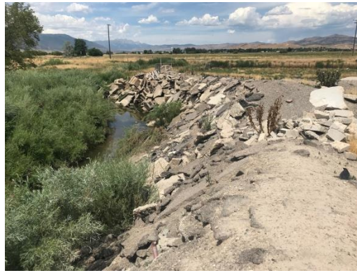
Illegal Fill Near Moroni
